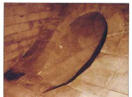
Fig. 7: Entry zone, tangential nozzles
